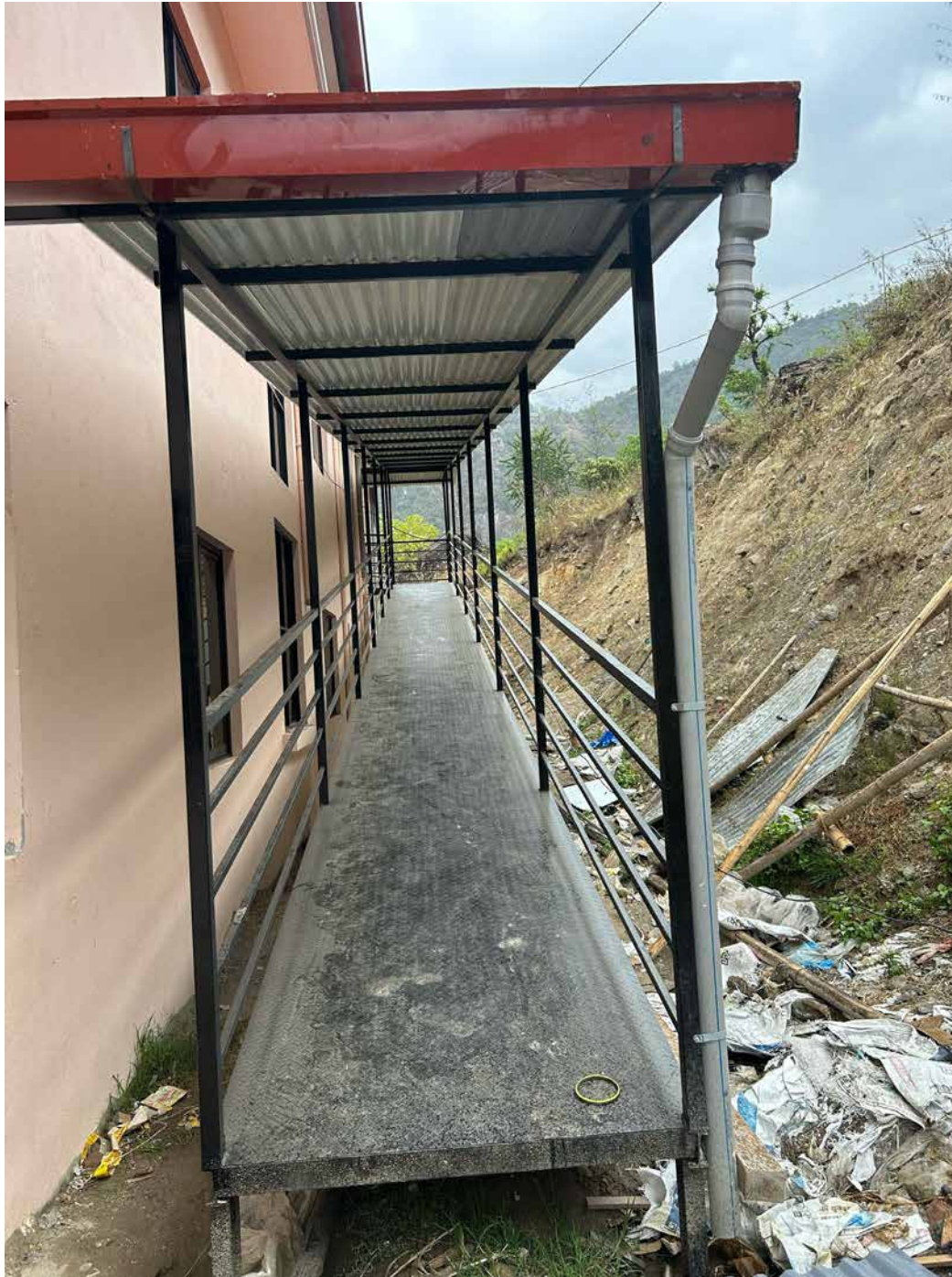
Wheelchair access ramp.
